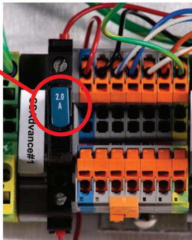
Figure 2.4 - DC Power Distribution
