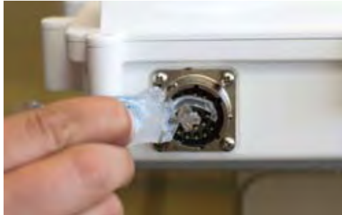
Figure 1.6 – Applying Silicon Dielectric Compound
