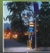
Solar General Lighting
